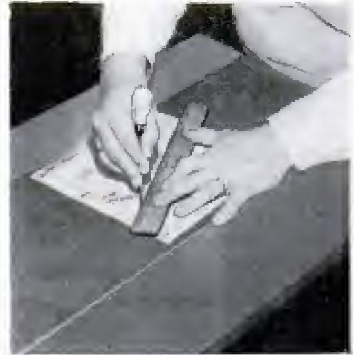
Asphalt tile can be cut by scoring on both sides with an awl, then snapping sharply
